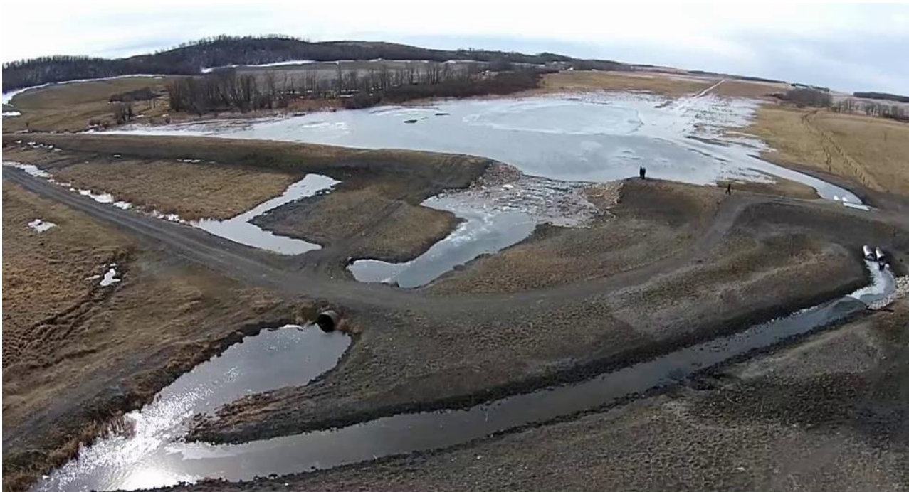
Figure 2. Aerial view of the Pelly's Lake Water Management Project in operation retaining spring runoff water (20 March 2015). Wetland habitat extends to the horizon, areas of harvested cattail in the deepest section closest to the earthen dam is fully under water. Opening of the gated culverts (right side of photo) will lower water levels allowing new wetland habitat to emerge. The ability to control water levels allows for autumn harvest of biomass.
