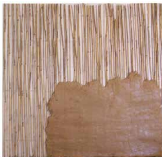
Figure 19. Sample 9: plastering in progress.
