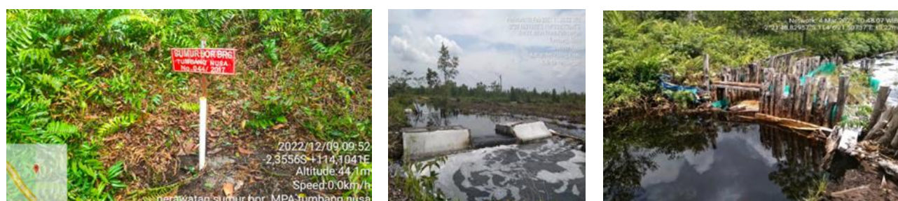
Figure 8. Deep well (left); canal blocks using concrete material (centre) and timber/logs (right).
