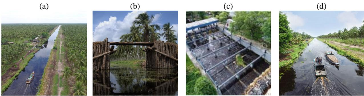
Figure 2. The three components of the water management system: (a) canal, (b) dike, (c) water gate, where (d) the canals are used as the main transportation system in the area.
