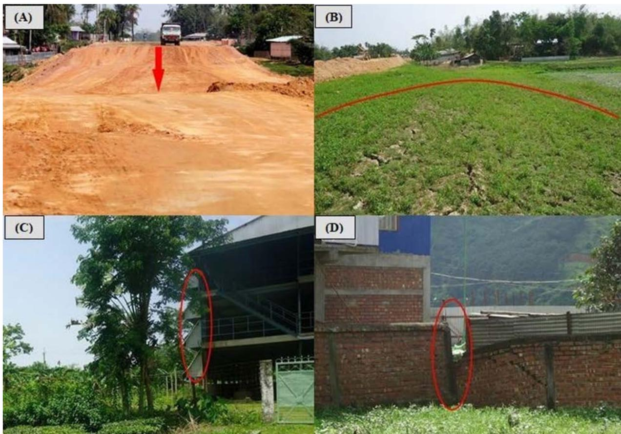
Figure 1. (A) and (B): embankment subsidence followed by heaving and shrinkage of adjacent ground at National Highway 39 (NH39); (C): a tilting building on peat at Kalinagar Tea Estate (KTE); (D): an existing structure sinking into the soil near the campus of National Institute of Technology, Manipur (NITM).
