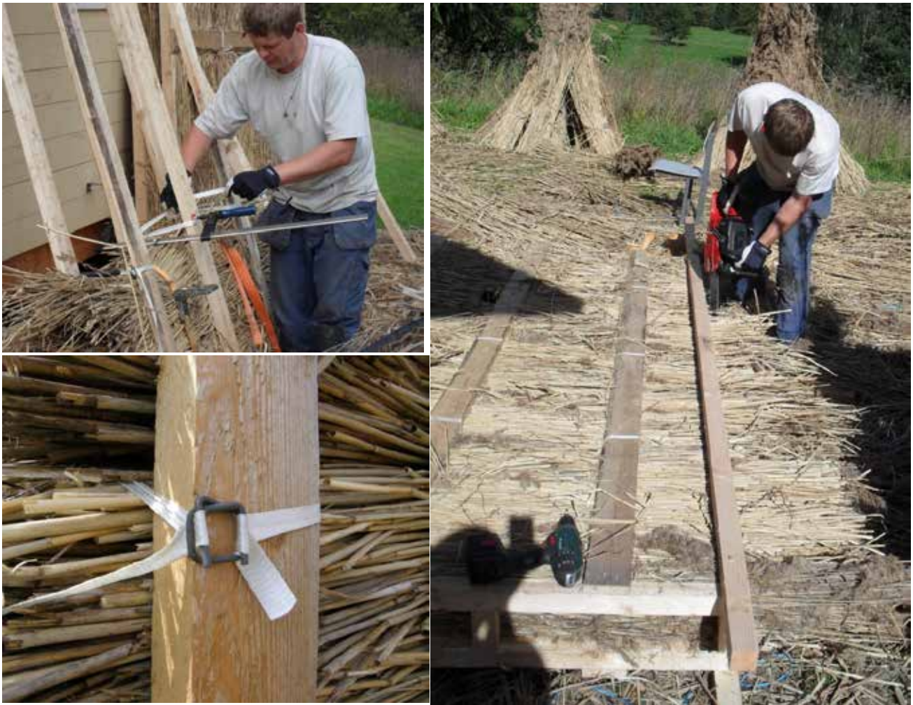
Figure 5. Stages in the manufacture of reed panels for Wall VS3. The timber frame was filled with loose reed by placing the stems horizontally, compressing and tying them to the frame posts (left), then trimming with a chainsaw (right).
