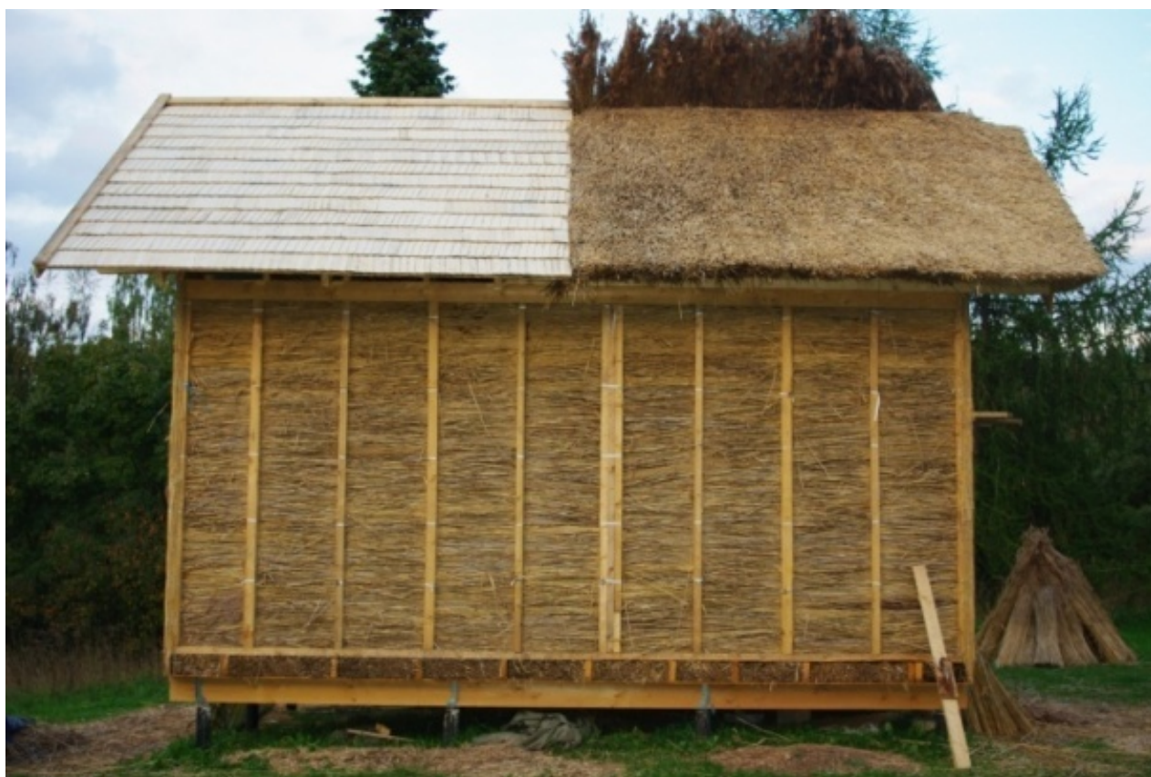
Figure 3. Photographs of two walls of the test house during construction. Above: wall type VS1 (with reed laid vertically); below: wall type VS2 (with reed laid horizontally).
