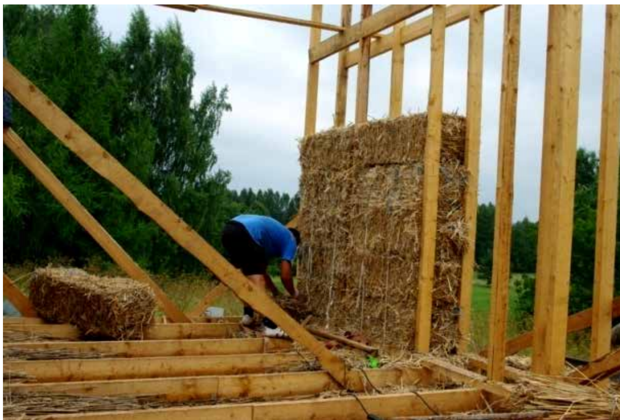
Figure 7. Photographs of two walls of the test house during construction, before rendering with clay plaster. Above: Wall VS3 (reed panel wall); below: VS4 (reed block wall).
